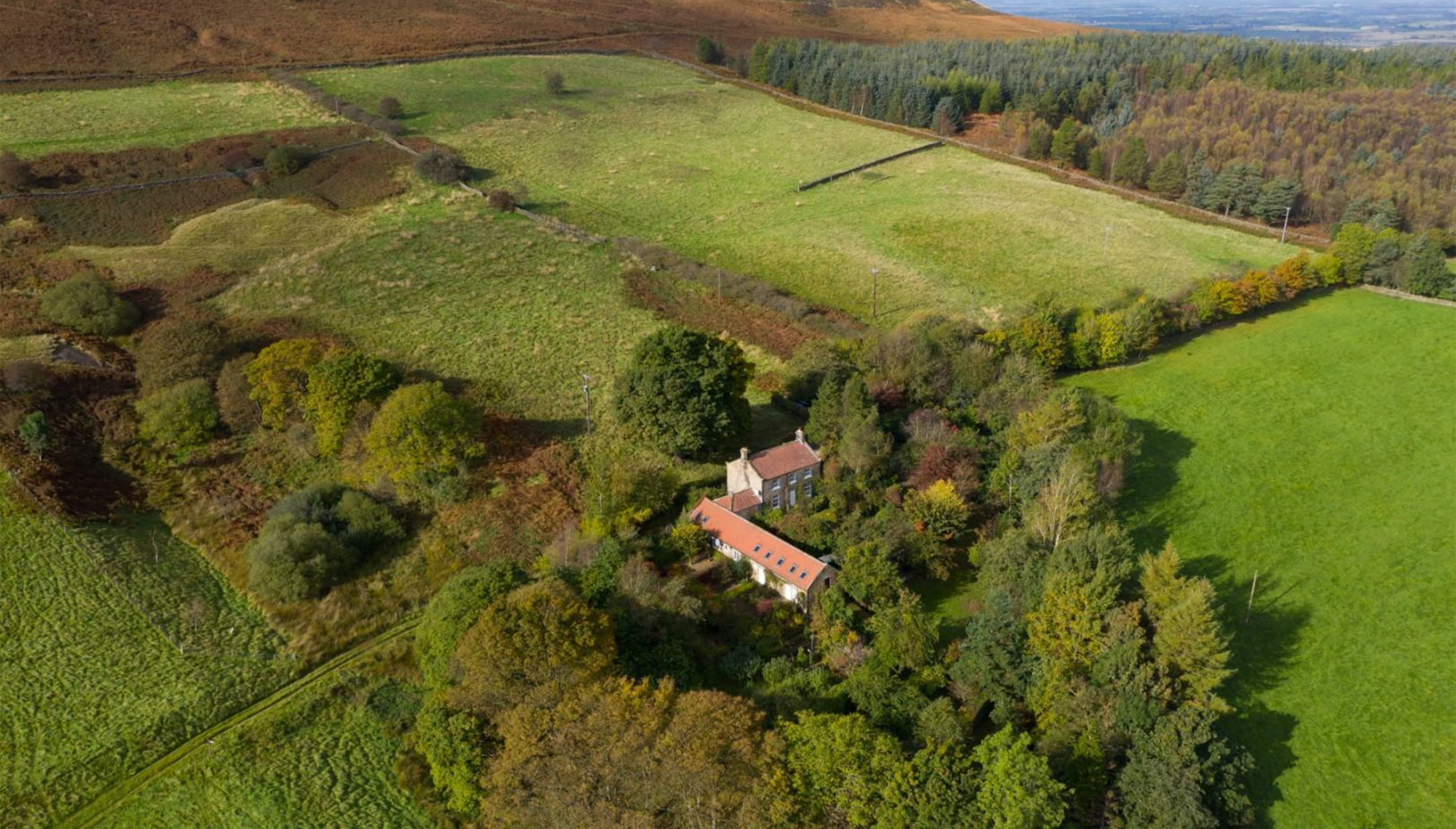
Thwaites House | Chop Gate, North Yorkshire
